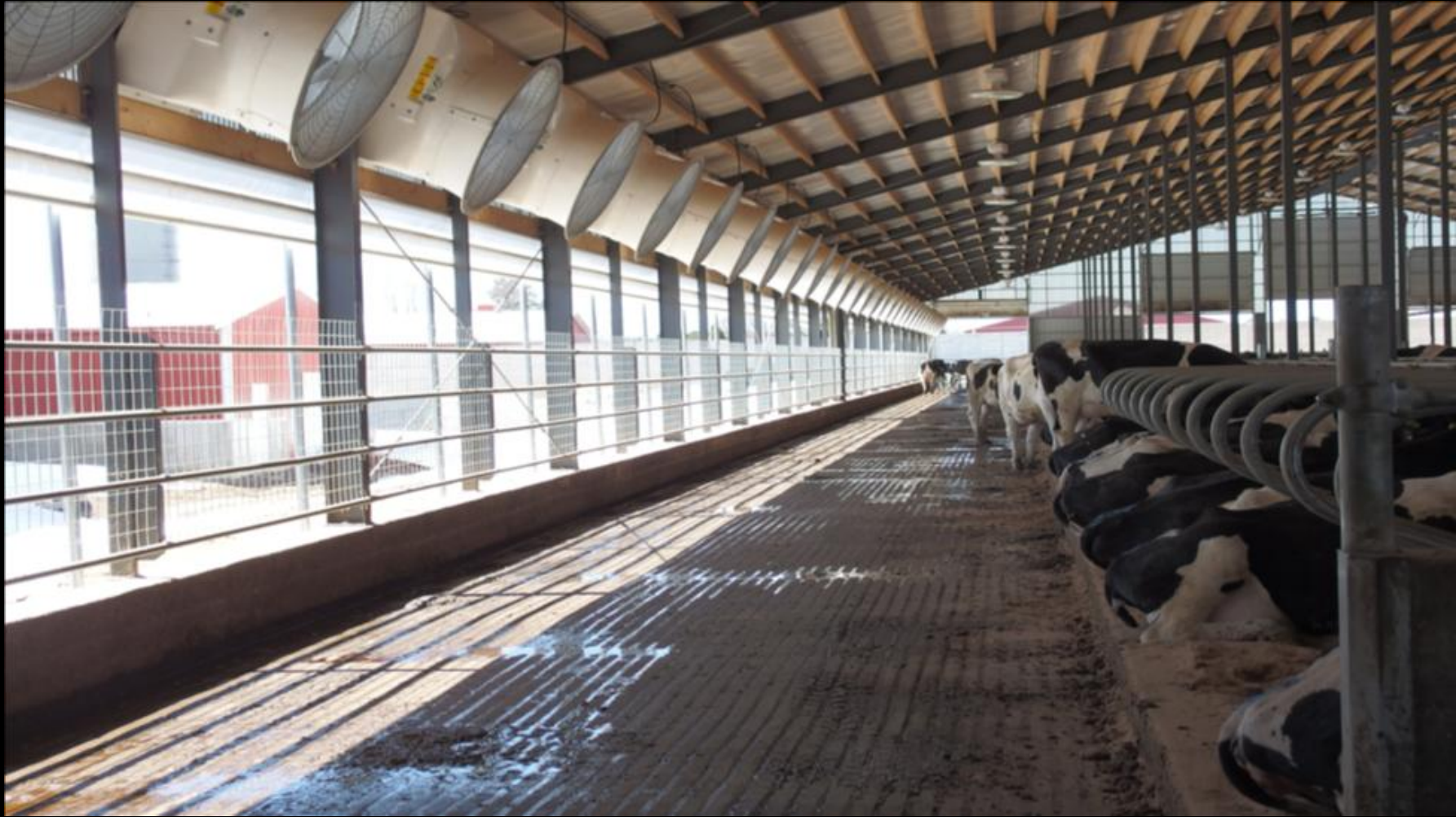
Positive pressure hybrid ventilation (Gordon Jones)
